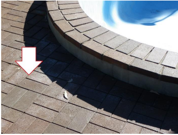
Figure 3 Dark pavers and coping with efflorescence present, with drainage. Resulted in blisters on pool walls.
