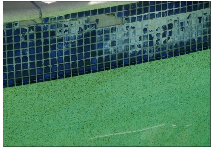
Figure 4 So many water related issues resulting in tiles being pushed off. Note area below tiles seems fine, as being porous.
