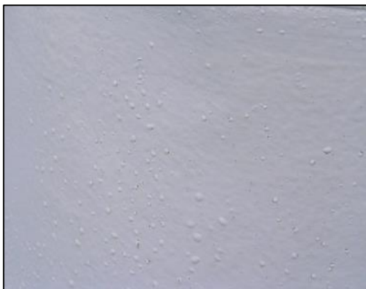
Figure 5 Painted wall showing hydrostatic blisters
