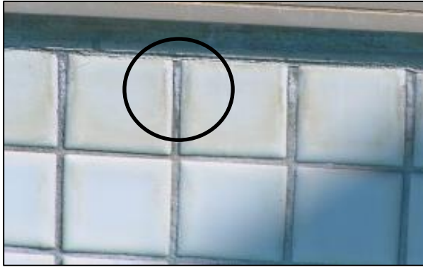
Figure 3 Showing telltale efflorescence on tile grout indicating water passing out from pool shell.
