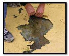
Often some areas of fiberglass will come away easily and others will remain very hard to remove, if at all. Usually, it will be necessary to remove the fiberglass where possible and replace OR feather edge the bigger patches leaving clean, bear concrete, fill any remaining holes with epoxy and hope the remainder of the fiberglass that is currently well adhered remains so. Ideally, ALL fiberglass needs to be removed no matter how well adhered.
