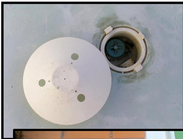
Fig 1: Typical hydrostatic valve assembly
