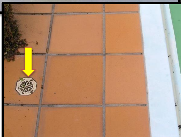
Fig2: A grating covering a tube near the pool to check the water table – level. (See arrow)
