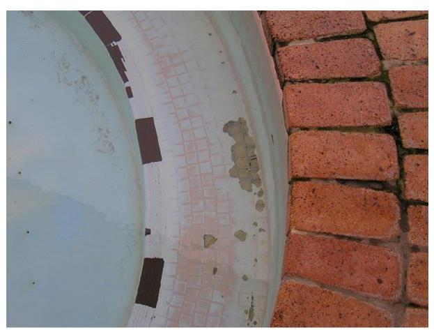
Ideally existing tiles, if generally okay, are best cleaned and re grouted as necessary. See a tile shop for suitable cleaners. Try a "lava stone" dipped in Calcium, lime, rust remover (CLR - Bunnings) as a rubbing and cleaning compound. Good results have been observed.
