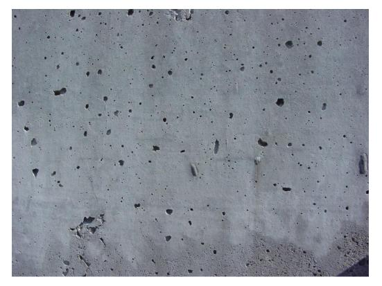
This system will fill these blow holes and indentations quickly and effectively leaving a smooth surface to coat. Suitable for fibreglass, concrete (bare or painted) surfaces. Just make sure all surfaces are clean and dry before carrying out this process.
