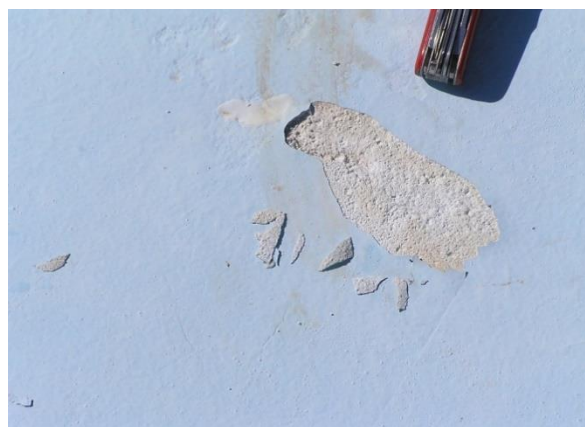
Fig 4: (above) The substrate failing internally and coming away, bringing the paint with it. Often due to hydrostatic pressure beneath and coming through the concrete shell.
