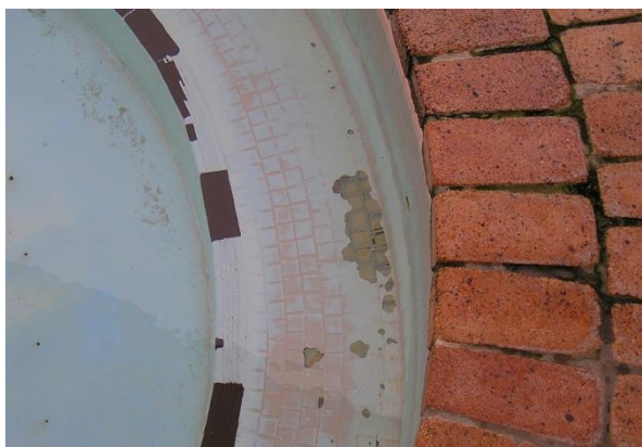
Fig2: (right) Painting of tiles is not recommended as it can lead to failure of the coating at the edges.
