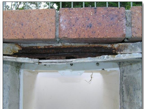
Check the metal plate above skimmer box
