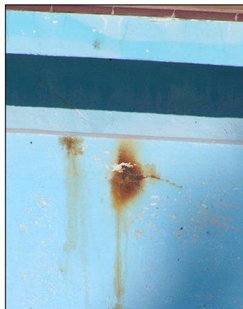
Crack with rust stains.
