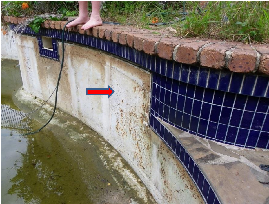
Pic 2 Depending on the shell construction upgrading with a coating is a better and much less expensive way to get the pool back into service. However , if the shell is of panel construction, then usually only an expensive liner can be reinstalled. Here we can see the panel joints (vertical lines) every metre along the wall, (arrow) meaning it probably can only have a new liner installed.
