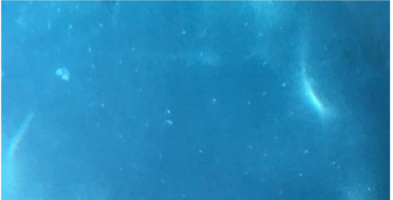
PHOTO: Thousands of tiny calcium nodules plagued this otherwise beautiful pool in a coastal town. Groundwater caused these, and the pool builder has since waterproofed every pool they build. No calcium nodules since.
