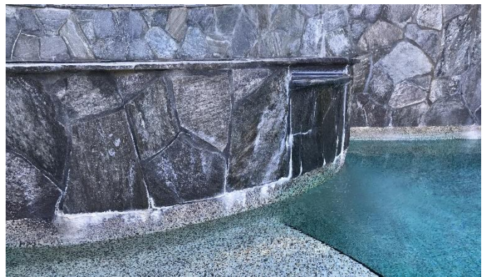
PHOTO: Efflorescence looks like carbonate scale because it is also calcium carbonate ( \text{CaCO}_3 ). But it is from moisture pushing through the concrete wall of the raised spa, taking minerals with it to the outside.
