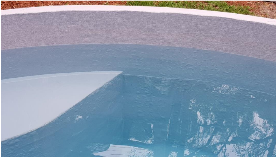
General view inside the plunge pool showing blisters above and below the water line.
