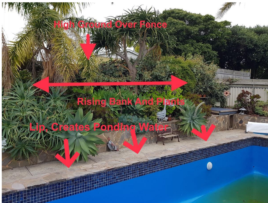
Image 2 Here is a pool with rising ground along one side (rises higher on neighbour's land) and combined with the rising bank and garden, is a great trap for rainwater and resultant seepage. (Into or under pool)
