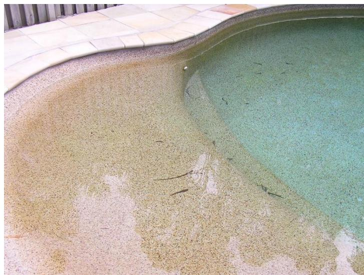
Pebblecrete is a cement and natural stone mixture trowelled over concrete and washed back to expose the small pebbles. Available in standard, mini, and polished pebble.
